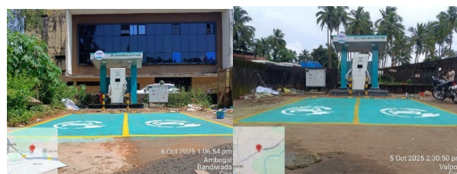
(EVCI installation work in progress at Goa Energy Development Authority (GEDA) locations)
